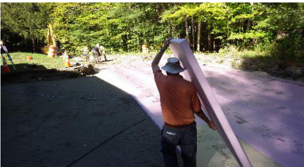
c. Placing insulation panels.
