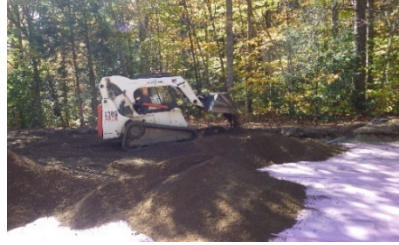
b. Spreading gravel base course.
