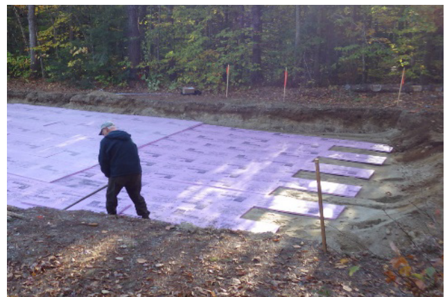
b. Panel insulation at site.
