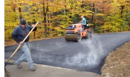
c. Rolling asphalt surface during construction.
