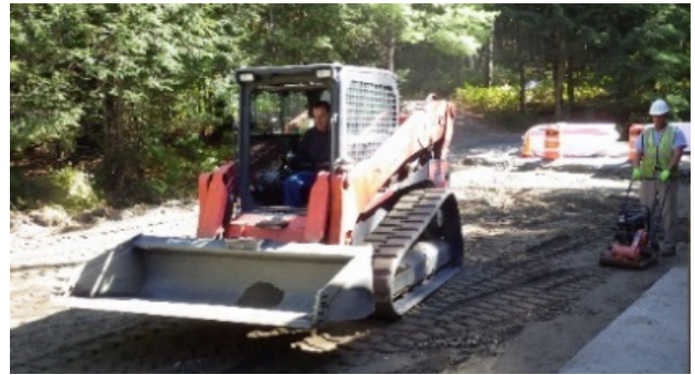
d. Compacting base course atop insulation panels.
